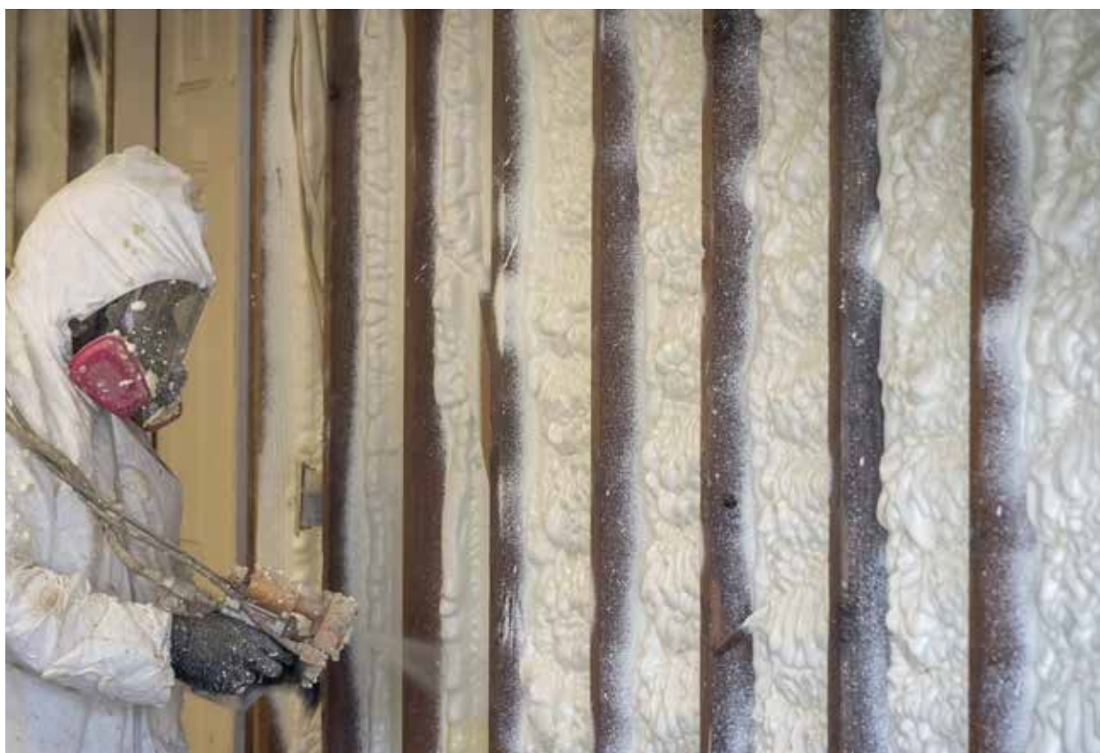
Right: application of spray foam
